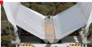
Gutters and downpipes
